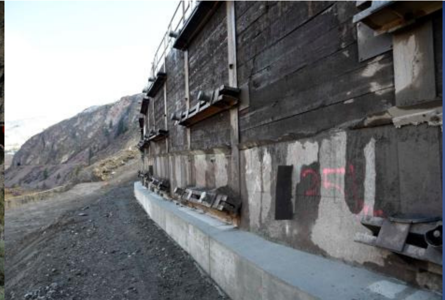
Fountain Slide – Retaining wall and slope stabilization
